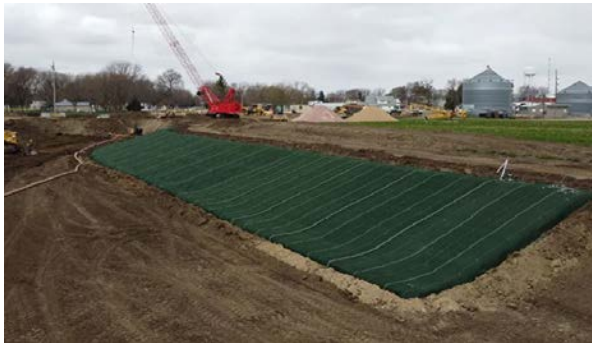
Figure 5 – Geosynthetic Mat Installed
