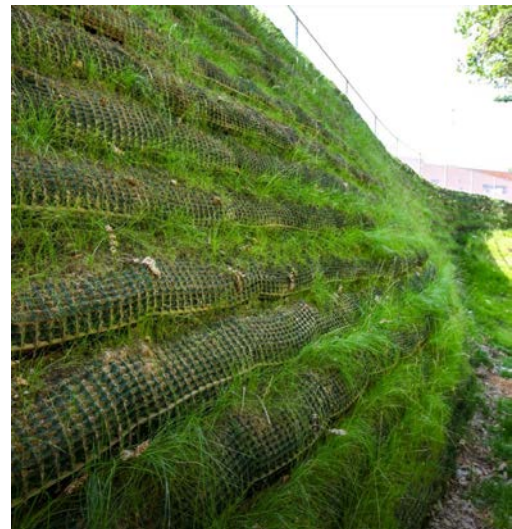
Figure 9 - Wrapped-Face Geosynthetic Reinforced Slope, Installed
