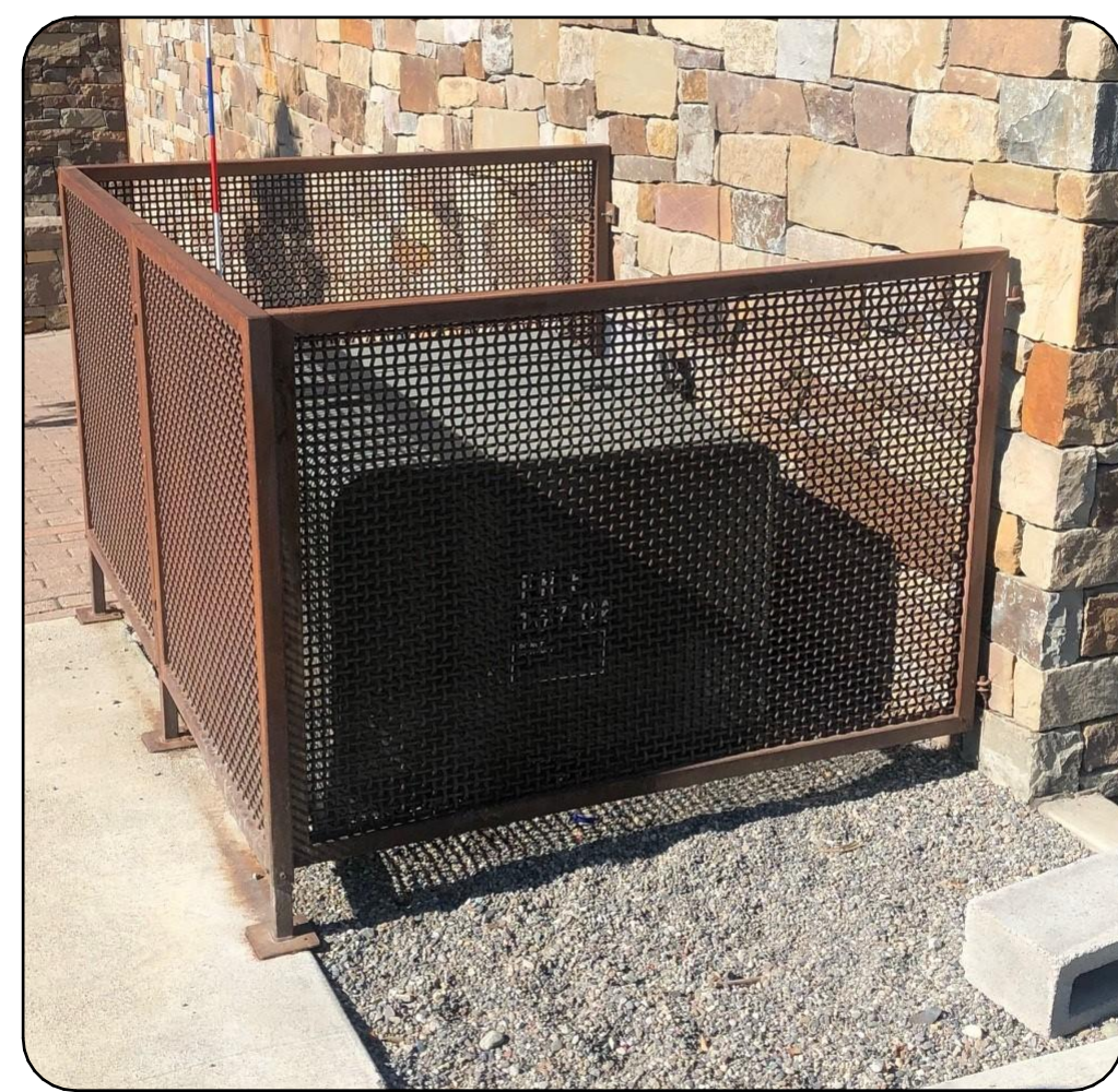
PHOTO: TRANSFORMER COVER EXAMPLE
