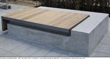
CONCRETE PLINTHS WITH INTEGRATED WOOD DECKING
